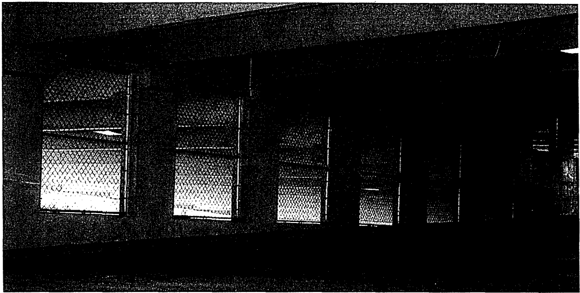
Figure 3-19: Image of the center wall of the prototype garage (Bayreuther, 2006).
