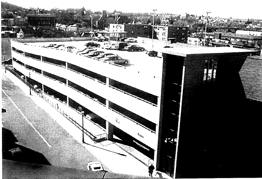
Figure 3-2: Lehigh University Campus Square parking garage (southeast corner) (Bayreuther, 2006).
